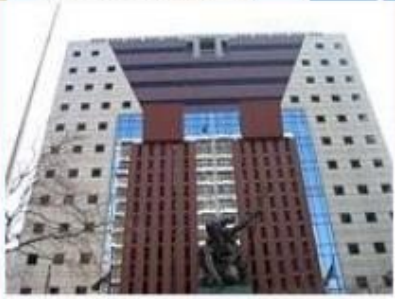
Portland Public Service Building Michael Graves 1982
